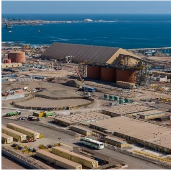
QB desalination plant.
